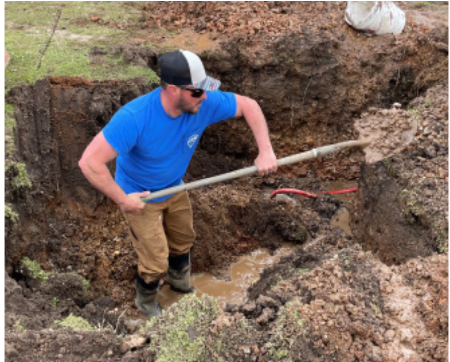
“Pokey” digging out a waterline to make repairs at the Woodlands.
