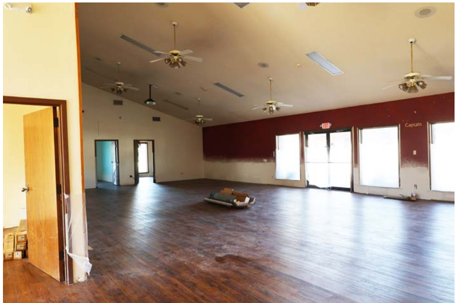
Progress continues at the BlueJacket Building.
